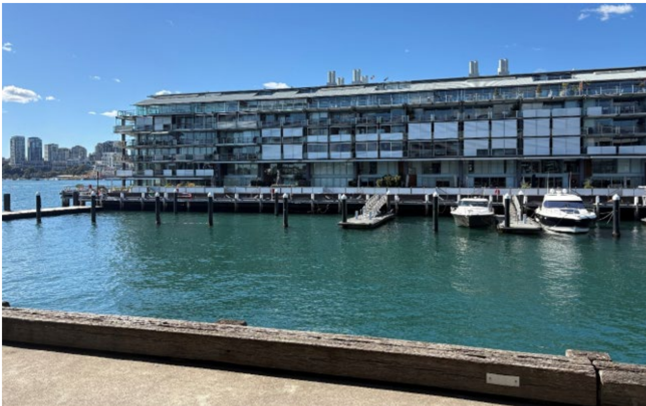
View of Pier 7/8 from site looking east
